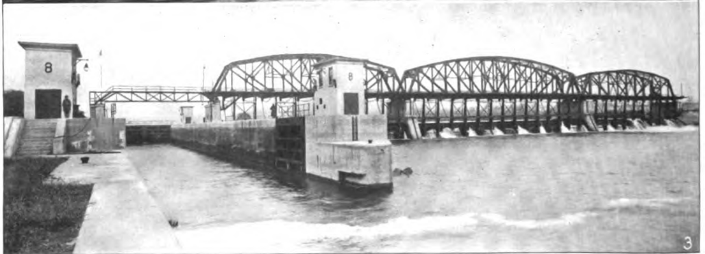
1 A dam 1,100 feet long and 100 feet high, forming a reservoir on Mohawk headwaters for supplying canal 2 Navigation of old-sized boats on typical river canalization 3 Lock and movable dam of bridge type in Mohawk river
